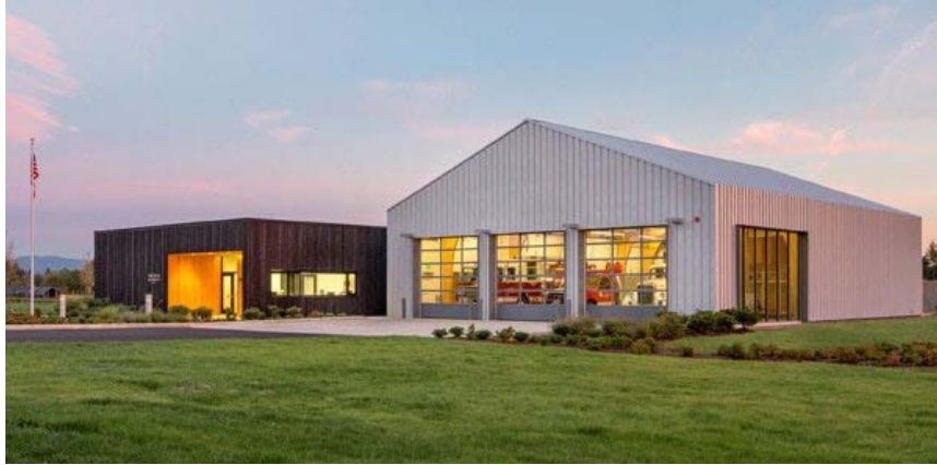
Owner: Multnomah County Rural Fire Protection District 10, Oregon Architect: Hennebery Eddy Architects, Inc Photo by Josh Partee
